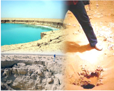
Stages of cavern collapse associated with subsurface dissolution
