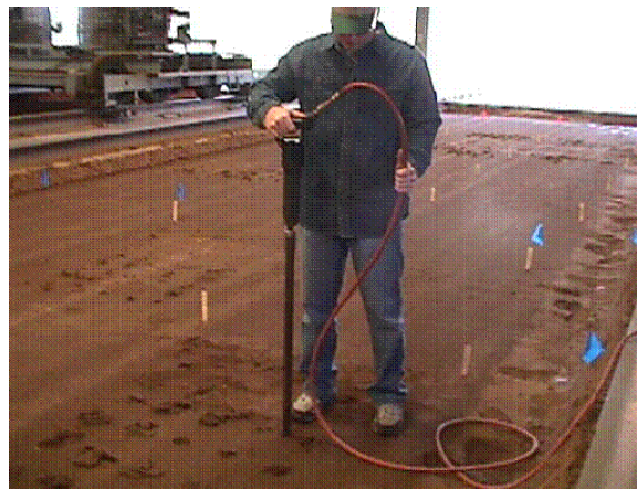
Figure B 2.8 Soil core sampling for soil moisture determination using air-jack hammer on the Norfolk sandy loam soil bin at the USDA-ARS- NSDL facility in Auburn, AL.
